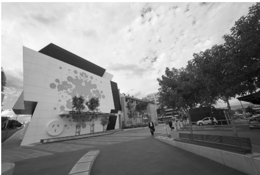
Figure 7: The PEP Dandenong conceived as urban 'space junk' with unknown functional logic dropped into the public plaza. Nervegna Reed Architecture. 2012. Photo Toby Reed
