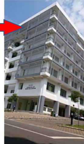
Figure 8 : Physical appearance of CADL ITB building. Source : Researcher, 2017
