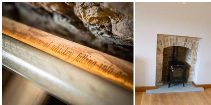
Figure 3 & 4. Timber handrail against exposed stair wall and first-floor fireplace. Source: Authors photographs
