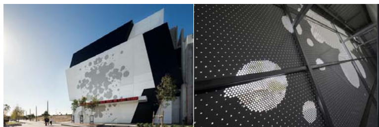
Figure 1: The PEP Dandenong exterior (L) and interior (R) has a perforated screen with optical black hole surface to the public plaza. Nervegna Reed Architecture. 2012 Photos John Gollings
